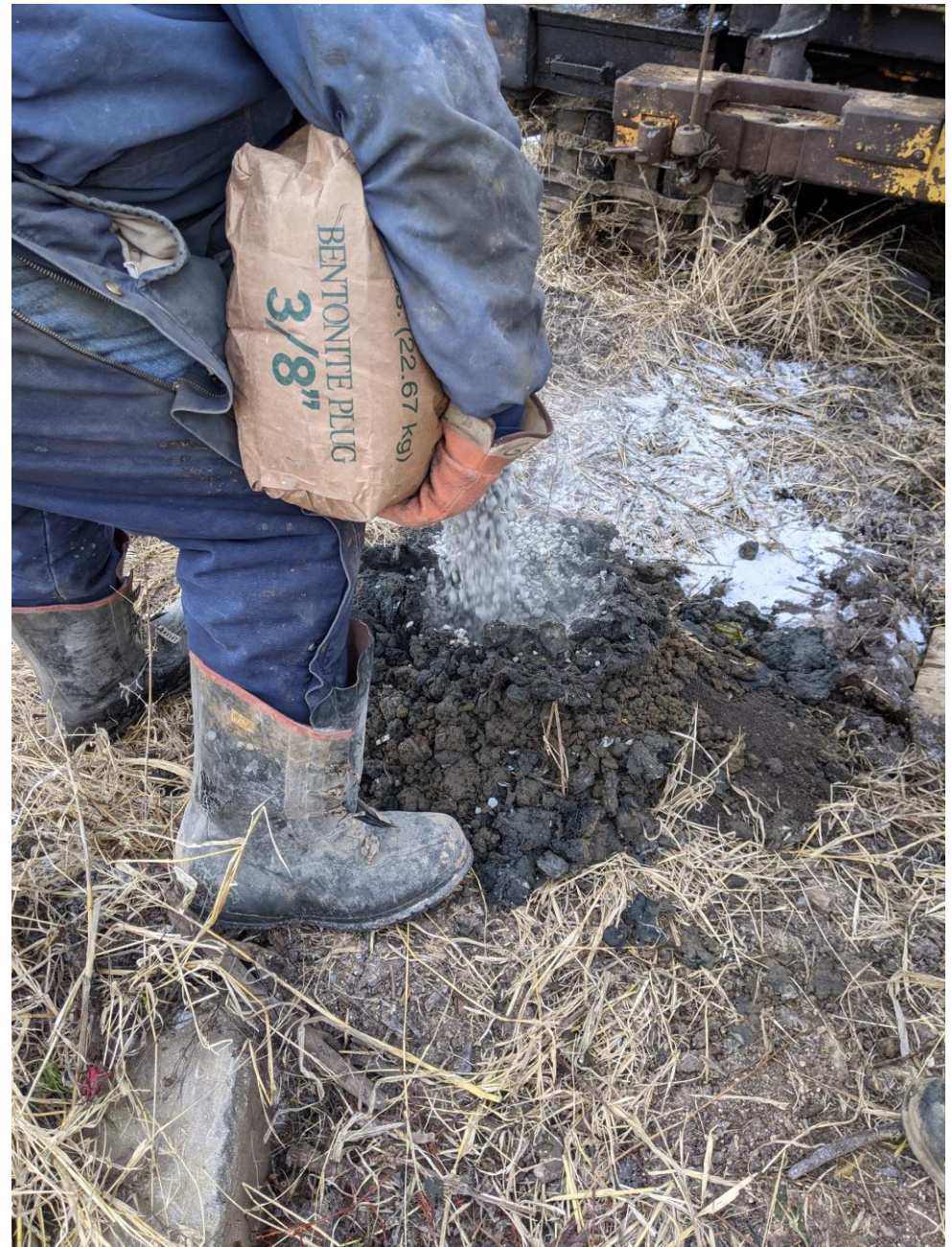
Right: B-3 being backfilled with bentonite chips after completion.
