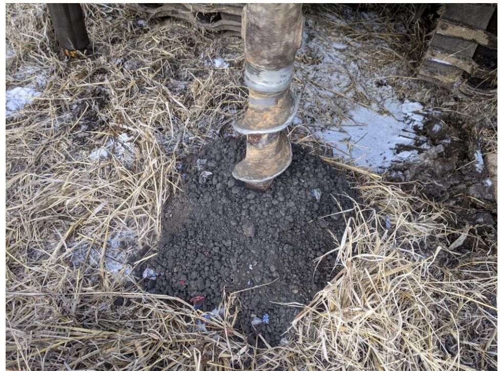
Upper right: Spoils containing deleterious material (plastic shreds).
