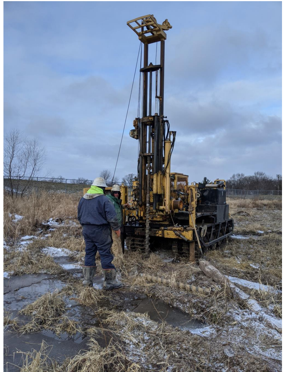
Right: Two-man drilling crew while drilling with hollow-stem augers between sampling intervals.
